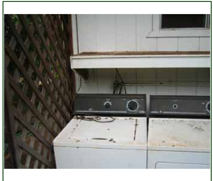
PHOTO 4: Leak at ohana washing machine faucet
