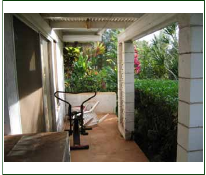
PHOTO 2: Rear patio slab and trellis
