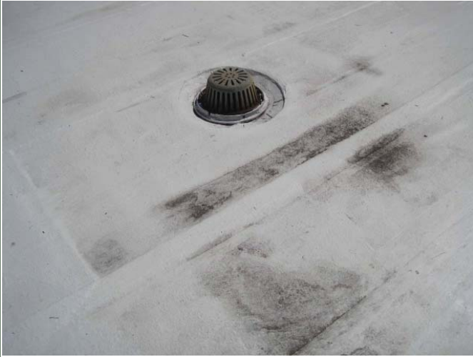
PHOTO 5: Possibly leaking roof drain
