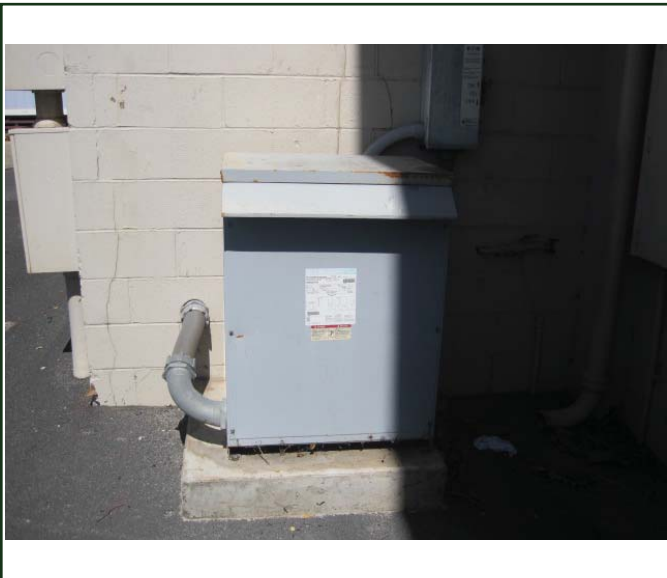
PHOTO 15: AC chiller transformer
