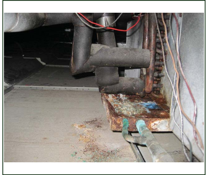
PHOTO 10: Corroded AC air handler, first floor ceiling
