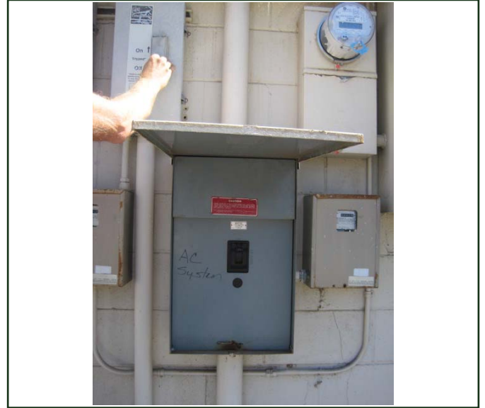
PHOTO 14: AC chiller disconnect panel
