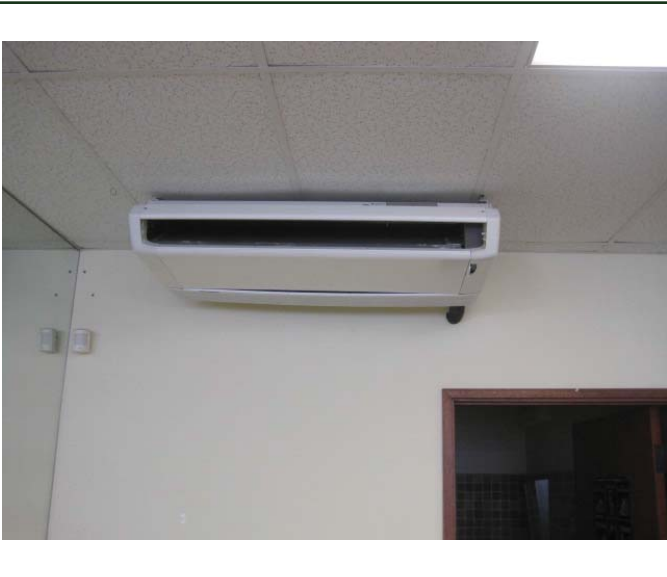
PHOTO 35: Abandoned split AC system
