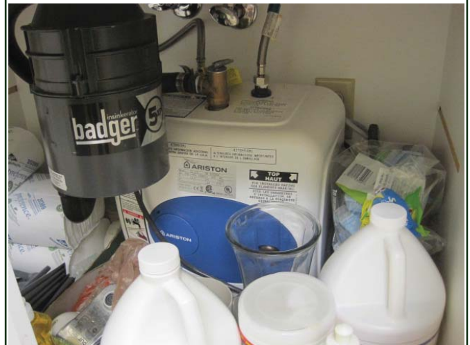
PHOTO 8: Ariston on demand water heater
