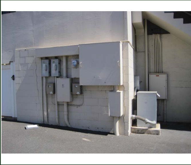
PHOTO 13: Main electrical meter and service panels
