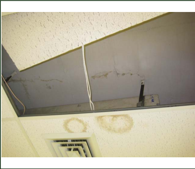
PHOTO 21: Upstairs ceiling tiles showing water damage and attempts at leak repair
