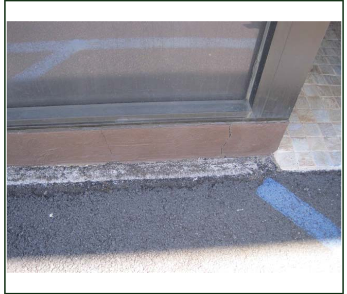
PHOTO 34: Spalling at front entry
