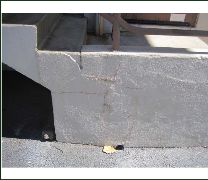
PHOTO 33: Spalling at rear steps
