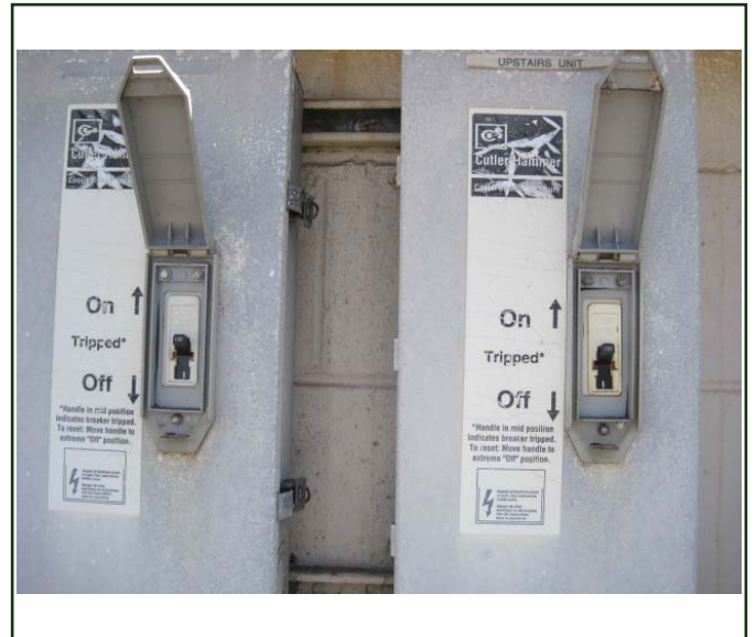
PHOTO 16: Interior power disconnects, one for each floor
