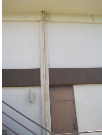
PHOTO 6: Possibly leaking roof drain downspout
