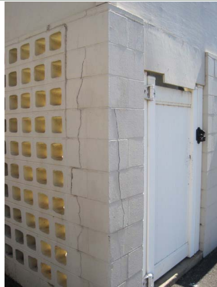
PHOTO 32: Spalling at AC chiller enclosure
