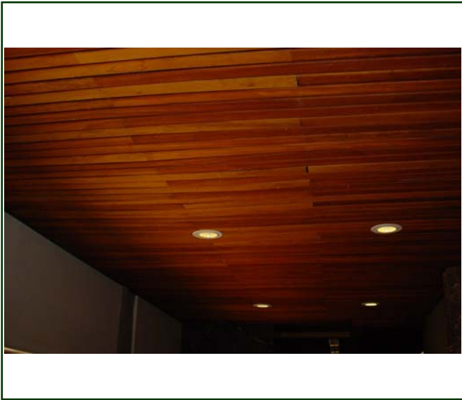
PHOTO 1: Corridor ceiling as seen on 1/6/2006
